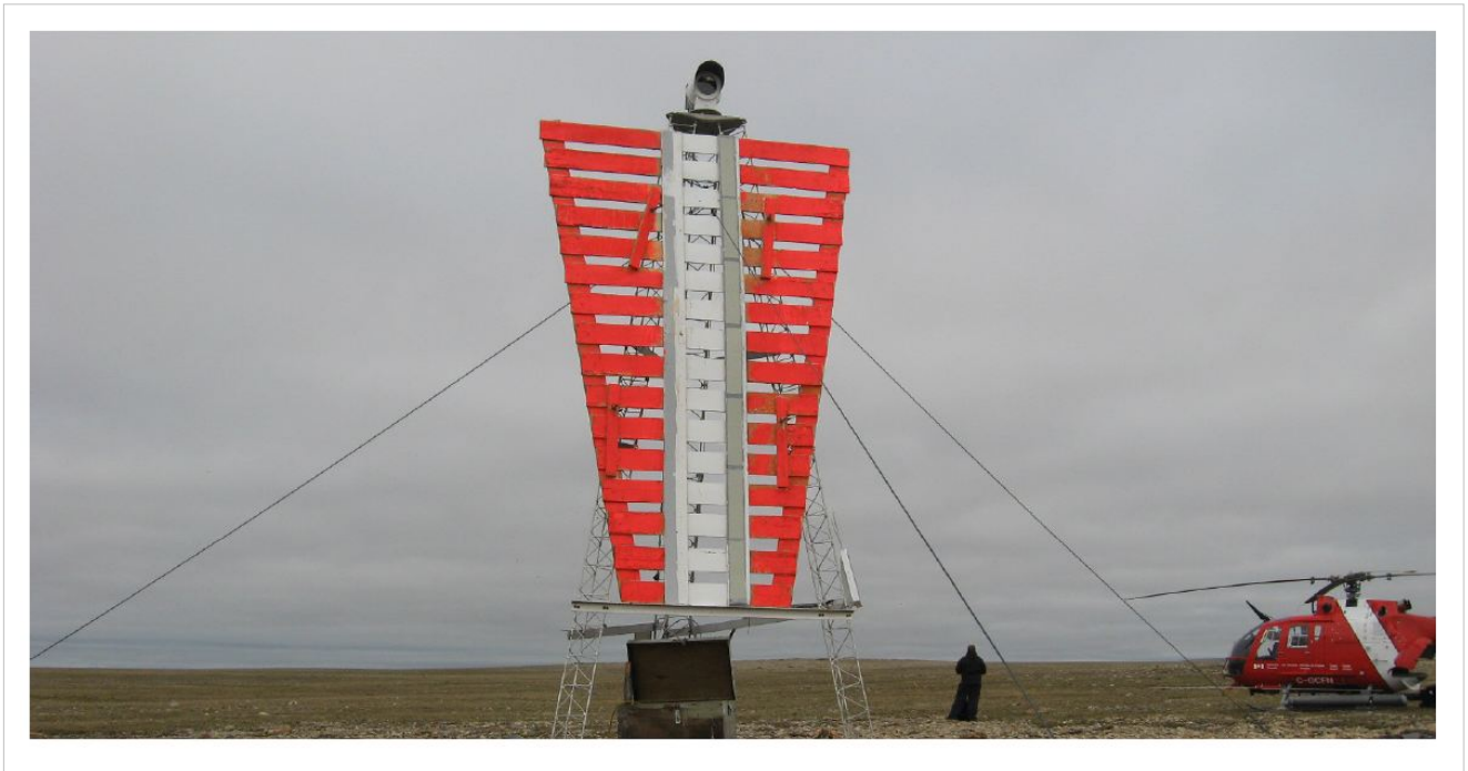
Leading (Rear Range) Light - Photo Courtesy of the Canadian Coast Guard
